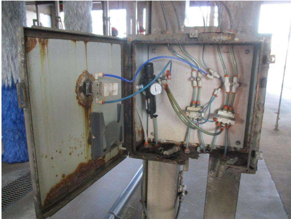
Existing Bus Wash Pneumatic System Metal Control Panel (e.g. pneumatic tubing, panel/cabinet, etc). Refer to contract documents for complete scope of work.
