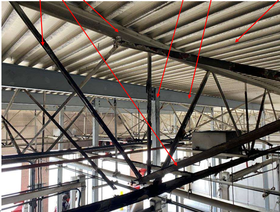
Temporary Roof Shoring
