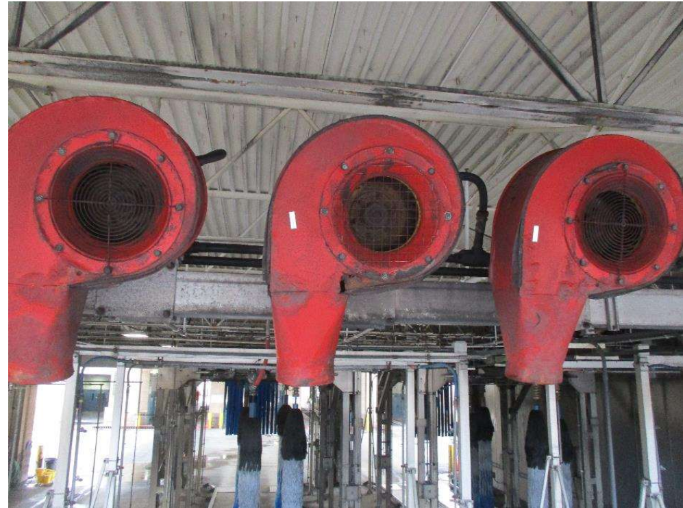
Existing Bus Wash Air Dryers (with corroded shrouds). Refer to contract documents for complete scope of work.
