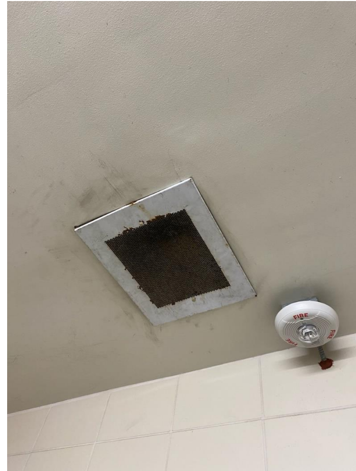
Typical Ceiling Mounted Exhaust Fan Unit at Men's and Women's Restroom
