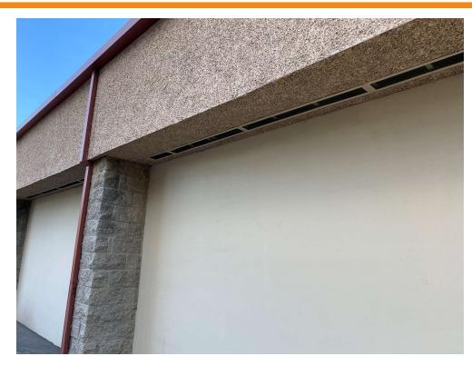
Various building components (e.g., soffit, columns, walls, metal gutter, metal downspout, vent grilles, etc.) subject to high performance painting and coating.
