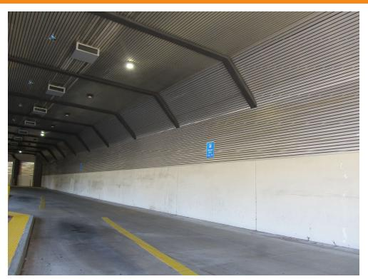
Tilt-up concrete walls and steel roof beams subject to high performance painting and coating; no new coating on existing aluminum ceiling. Refer to project plans for items to be protected in place.
