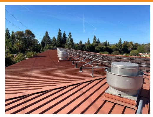
Metal roofing and metal roof screens subject to high performance painting and coating. Refer to project plans for items to be protected in place.
