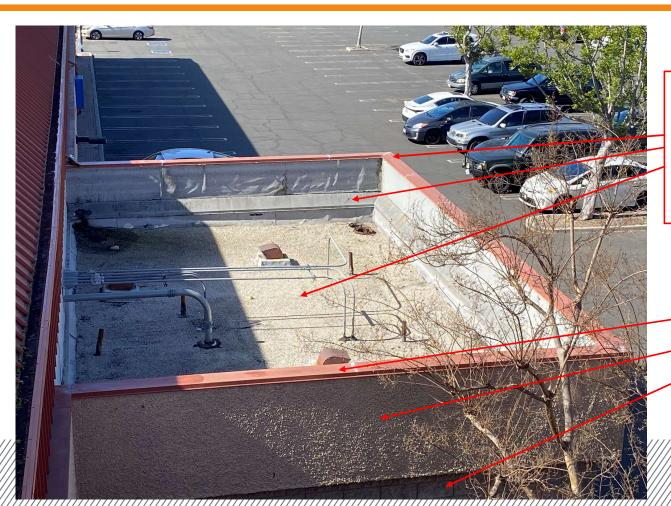
Existing restroom building roof system subject to be removed (and legally disposed of off-site) and to be replaced with new roof system. Refer to contract documents for complete scope of work.
