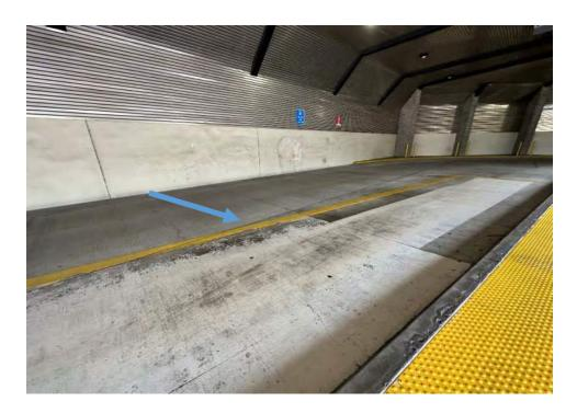
Photograph 4: View of the yellow traffic strip lead-based paint on the concrete road within the bus terminal.
