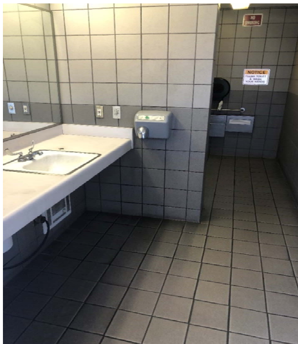
Photo 7 – Westerly Restroom Building, Drivers' Restroom
