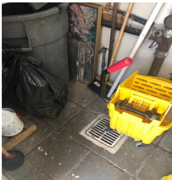
Photo 6 – Westerly Restroom Building, Storage Room with floor drain
