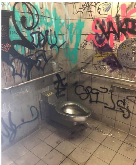
Photo 5 – Westerly Restroom Building, Men's Restroom
