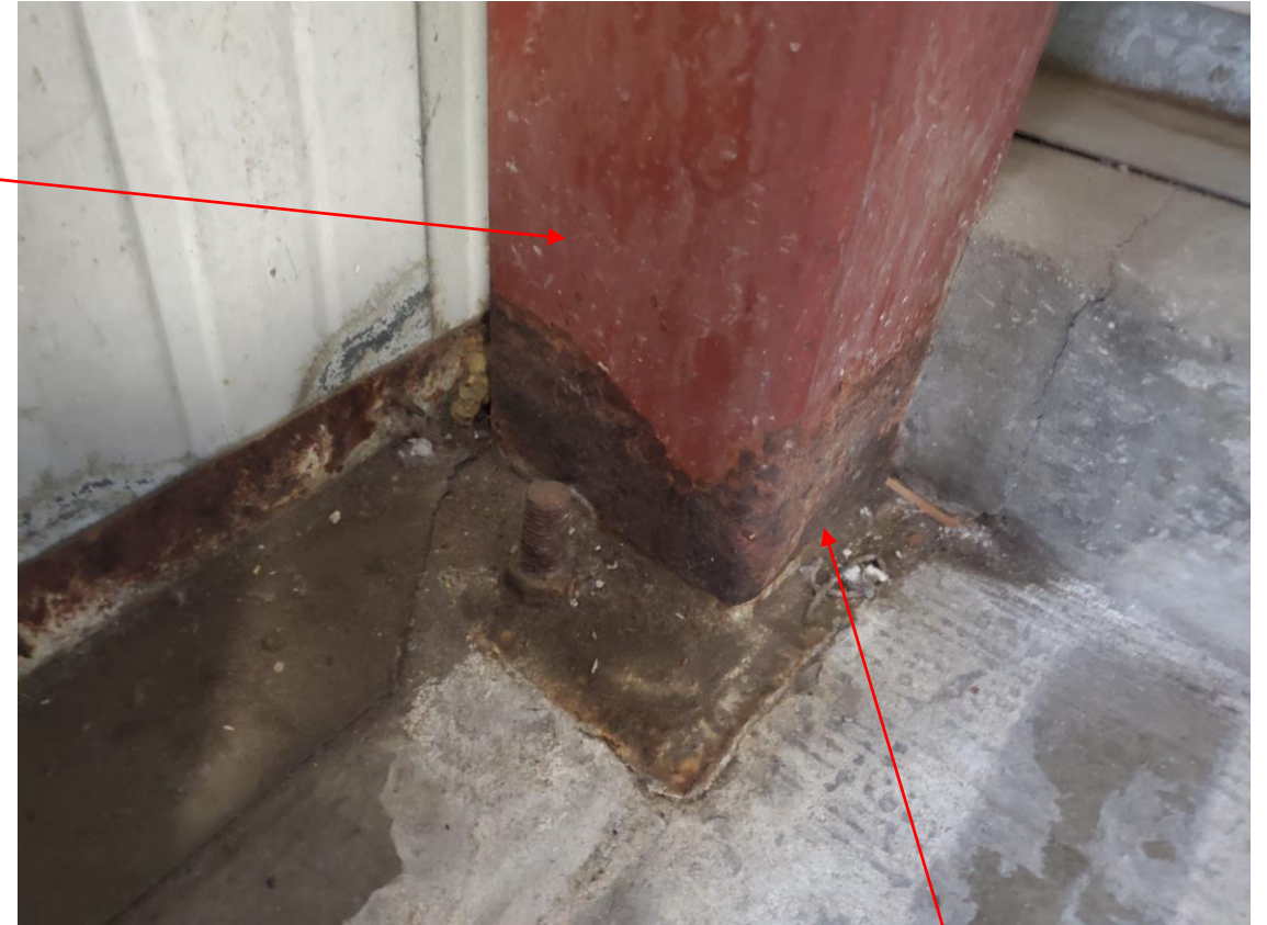
Rust at base of the columns
